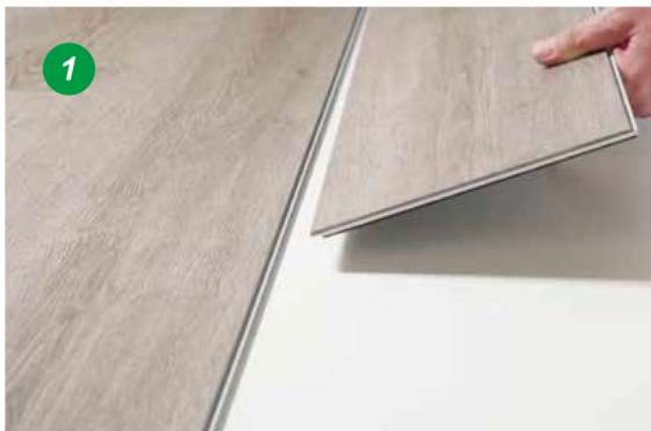
1 Connect the long side at an angle
