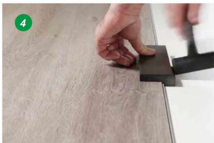
4 Use a soft-faced hammer to properly lock the planks
