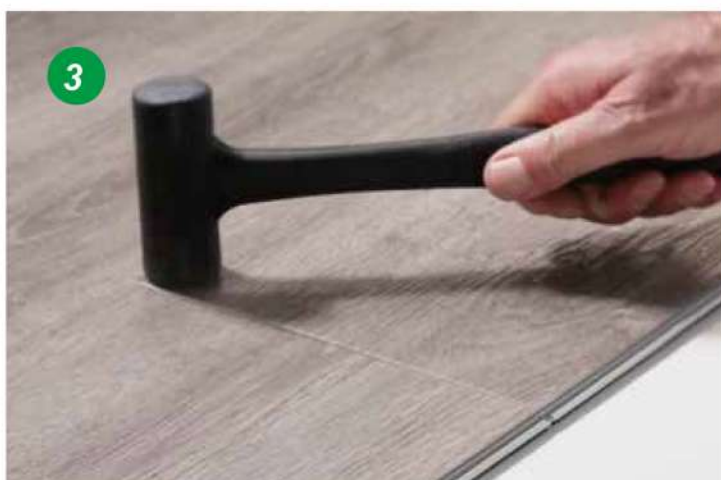
3 Use a soft-faced hammer to lock the planks on the short side
