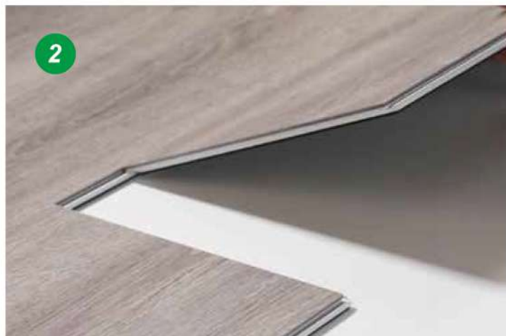
2 Slide until short side and drop
